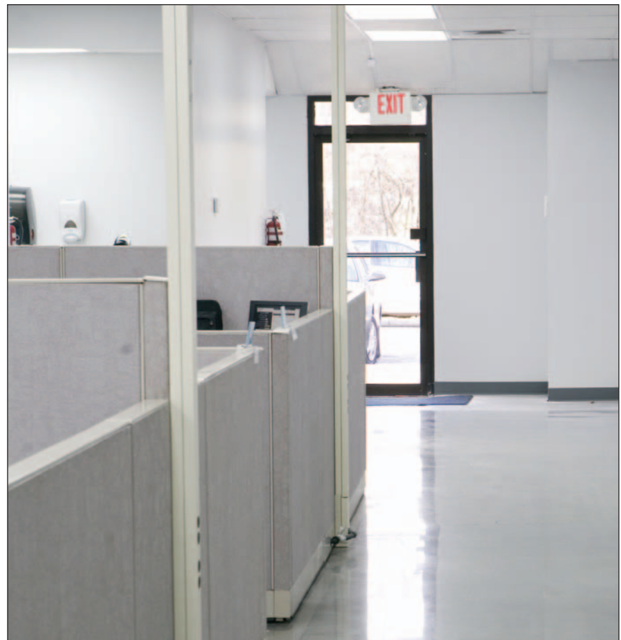
Light reflectance attained with a polish like this one can actually help save on lighting costs for office environments like the one above.
