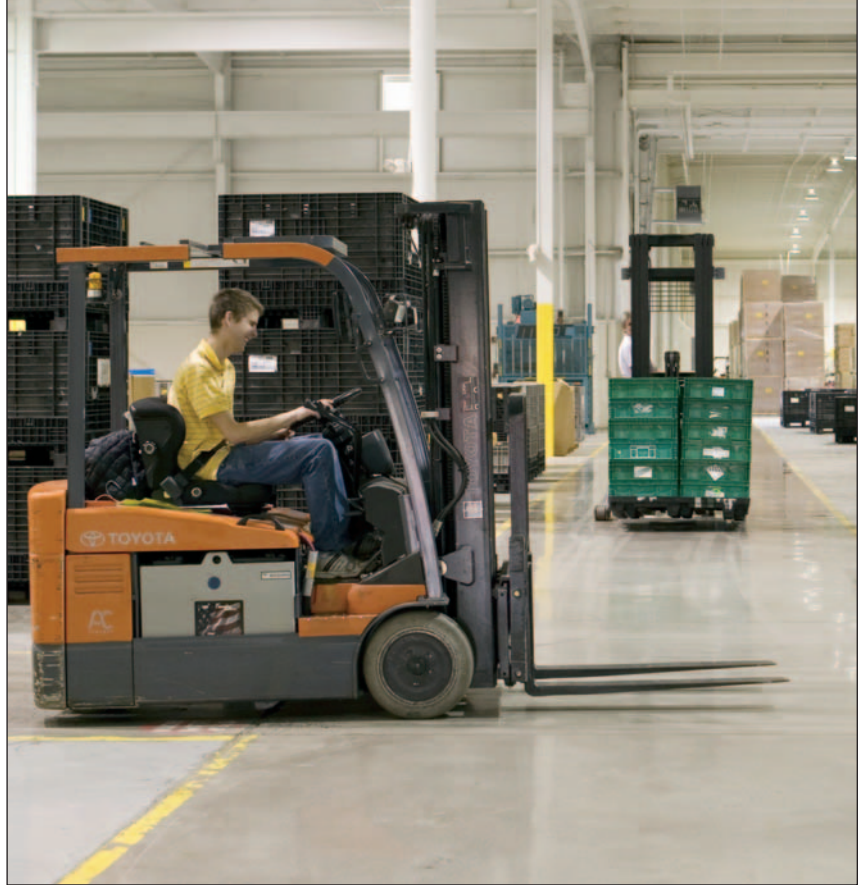
The light reflectance on this warehouse floor was attained by specifying polished concrete. Attaining the right shine depends on the number of diamond disc grinder passes.
